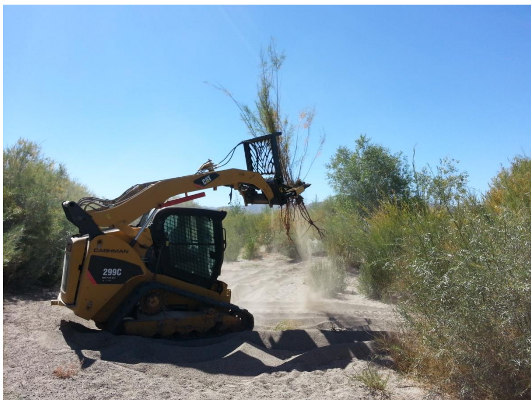
Mechanical removal of Tamarisk.
